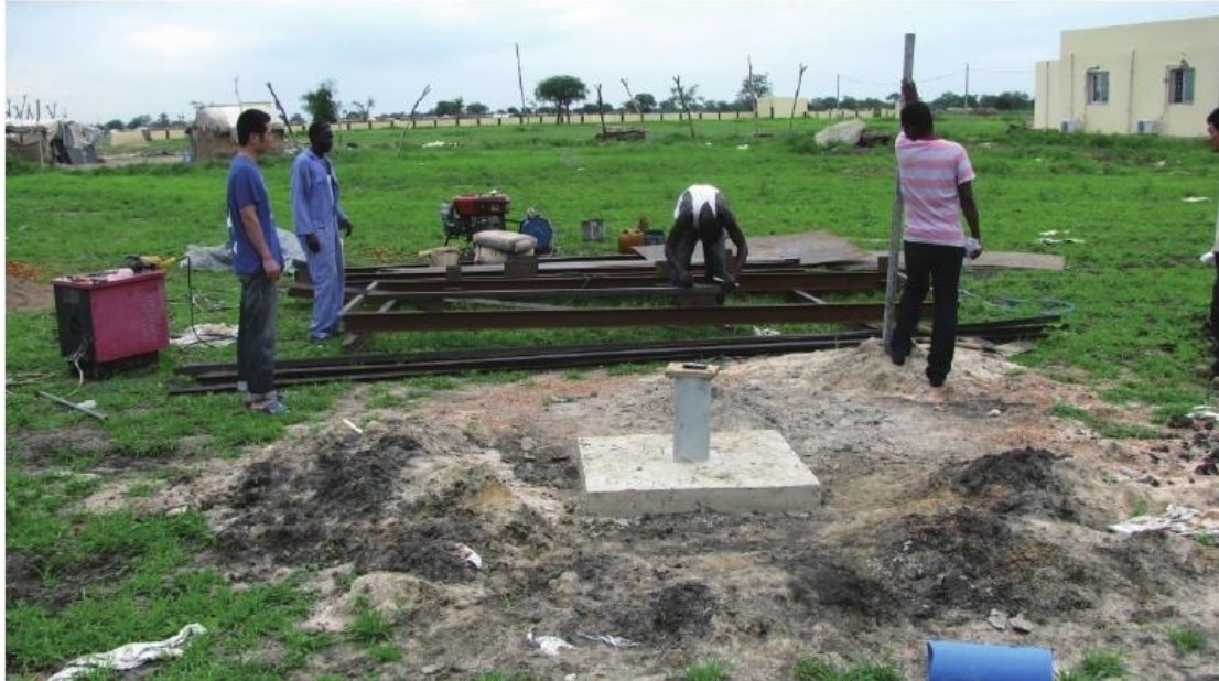
Fig. 4 Work-site of the municipal pipeline project, Abyei, Sudan
